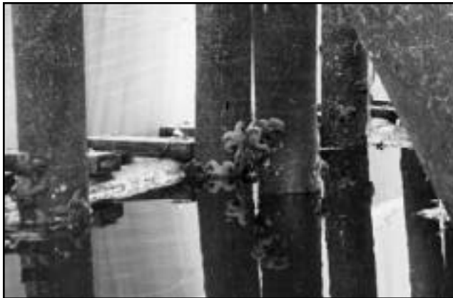
The piling were heavily encrusted with starfish, sea anemones, mussels and other varieties of sea life.
