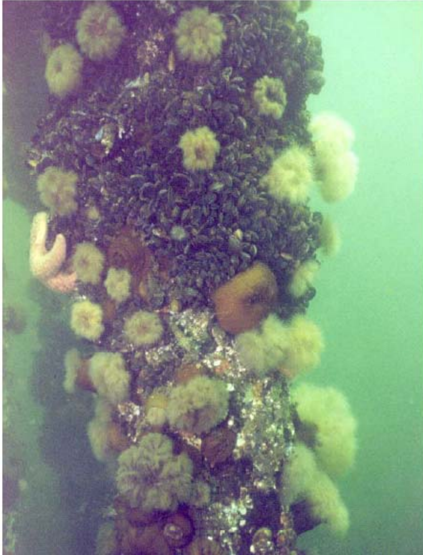
Sooke Basin Creosote Treated Piling After 4 Years In Place
