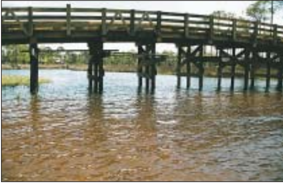
Horseshoe Bayou Bridge
