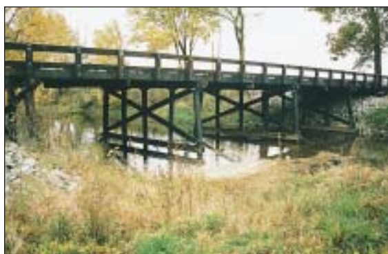
Pipe Creek Bridge
