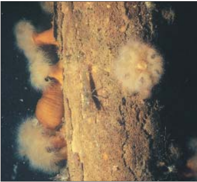
The untreated piling were deteriorating and did not support a vibrant fouling community
